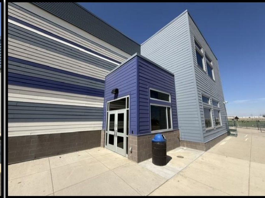
Primary – Vestibule Addition
