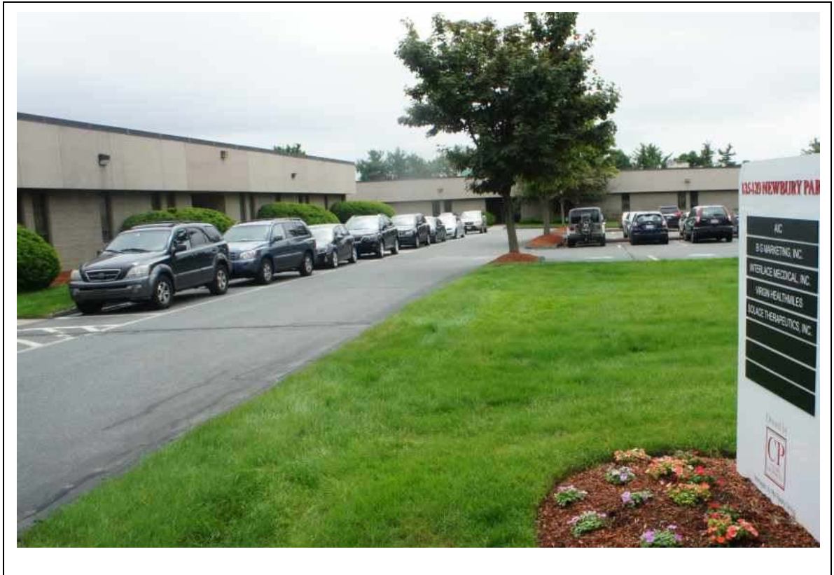
View of 139 Newbury Street, Framingham, MA
