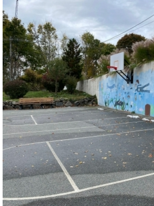
Exterior play space open to adjacent street is a security concern.
