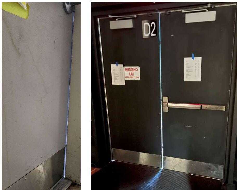
Daylight Visible Around Perimeter and Between Double Doors
