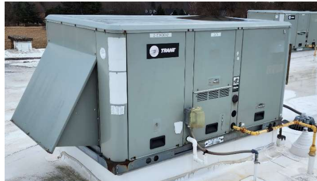
Typical RTUs Which Have Exceeded EUL
