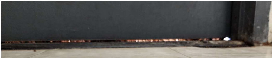
Typical Damage to Door Footers
