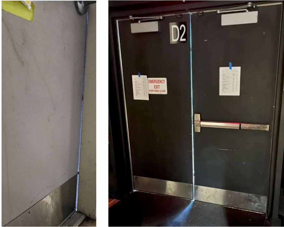
Daylight Visible Around Perimeter and Between Double Doors
