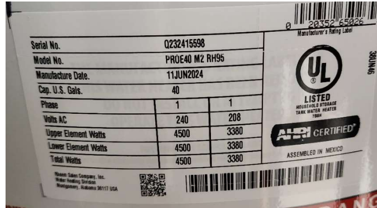
Chemistry Lab Hot Water Heater
