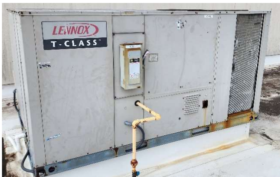
Typical RTUs Which Have Exceeded EUL
