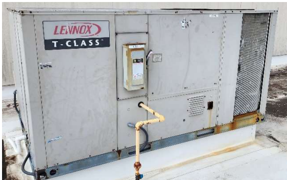
Typical RTUs Which Have Exceeded EUL
