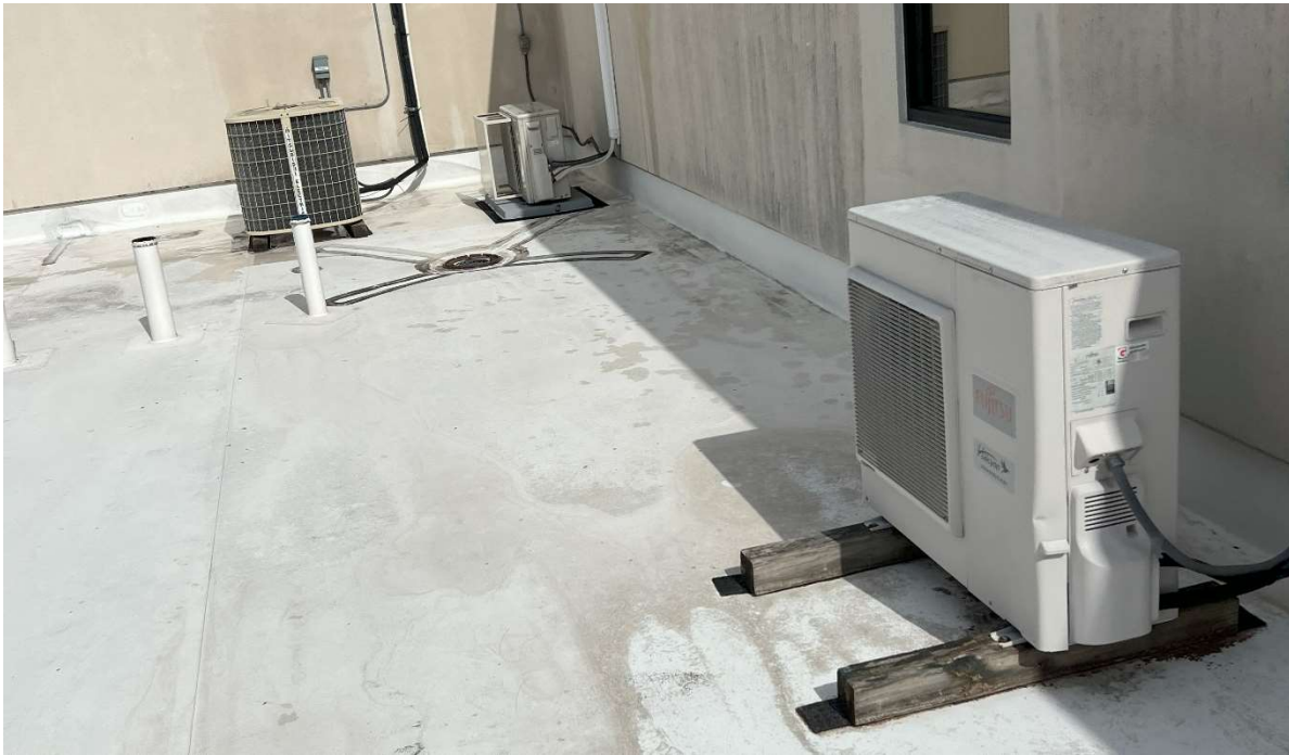
Split Systems Serving Computer Lab, IT Room, and 303
