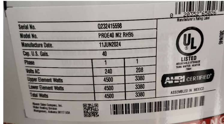
Chemistry Lab Hot Water Heater
