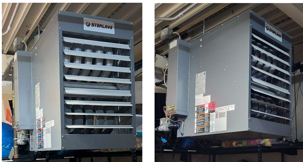
Typical Natural Gas-Fired Unit Heater
