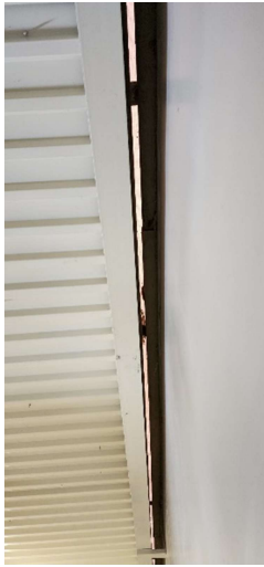
Unsealed Roof/Wall Line with Damage Due to Moisture
