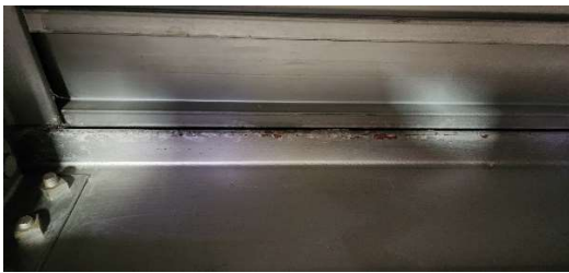
Unsealed Roof/Wall Line with Damage Due to Moisture
