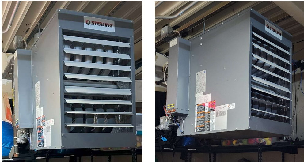
Typical Natural Gas-Fired Unit Heater
