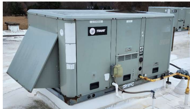
Typical RTUs Which Have Exceeded EUL
