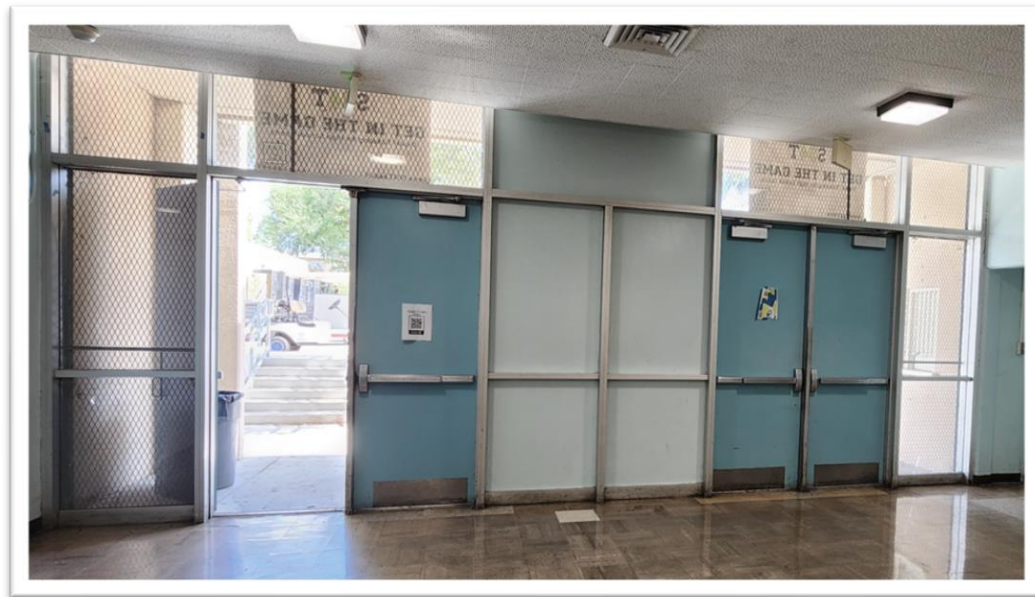
Image of existing door/window wall
