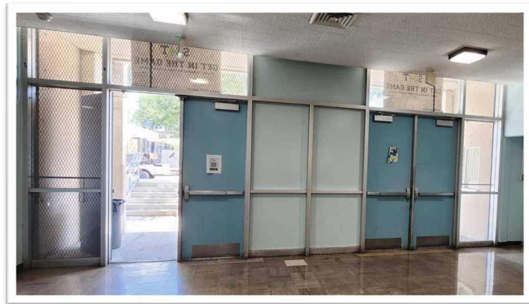
Image of existing door/window wall
