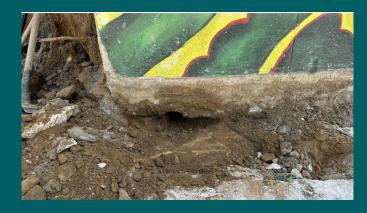
Recommendation: Ridgeline Construction recommends the demolition of the mural wall and having it re-built with proper support per structural engineers' recommendation.
