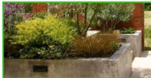
CAST IN PLACE CONCRETE PLANTER
