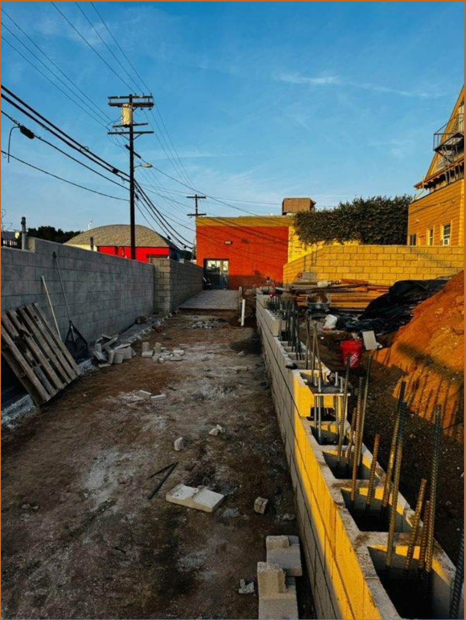
INCREASED BLOCK SIZE 12" WITH ADDED REBAR CORRECTIONS BY LADBS. PLEASE NOTE THE THE HEIGHT DIFFERENCE TO PARKING LOT ALSO REQUIRING ADDITIONAL SOILS ENGINEERING.
