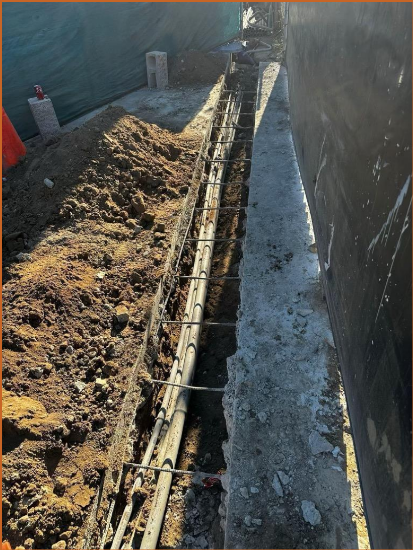
BRIDGE FOOTING REQUIRED TO SPAN THE METRO TUNNEL. REQUIRED DRAINAGE.
