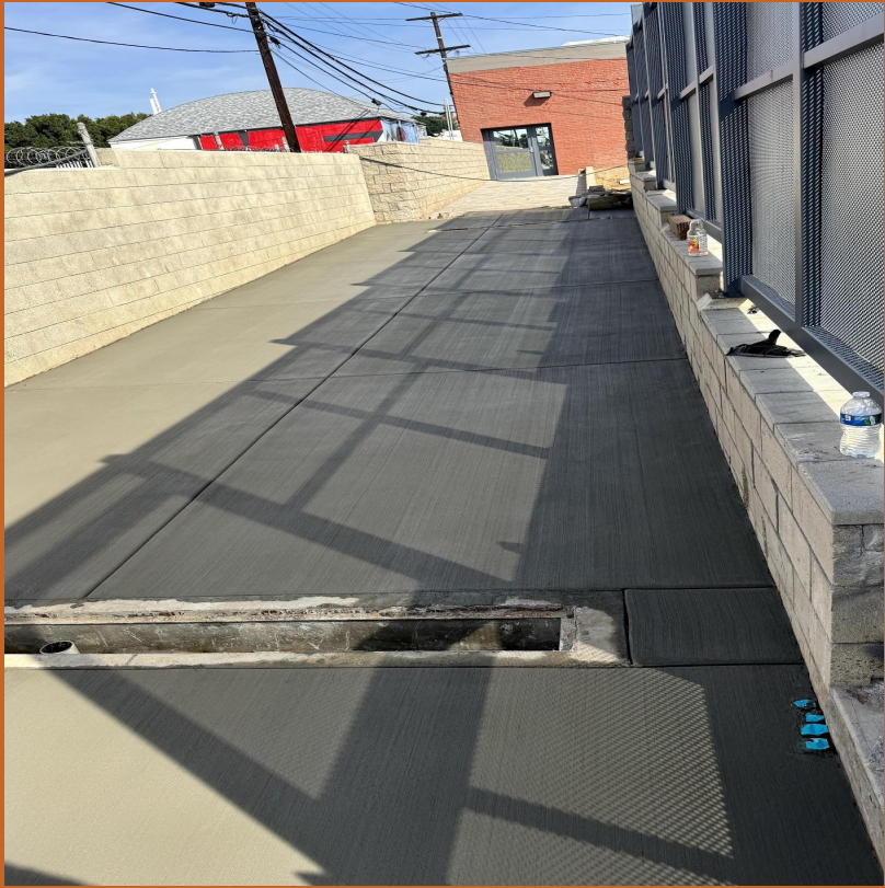
CONNEXION WALKWAY SHOWING DRAIN ROUGH IN. NEW FENCE IS INSTALLED.
