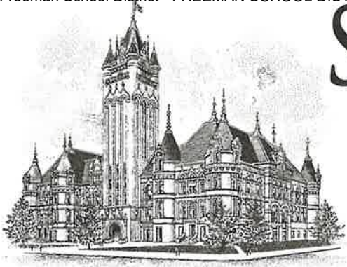
SPOKANE COUNTY COURT HOUSE
