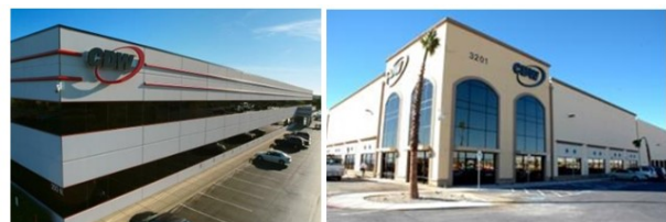
450,000-square-foot distribution center in IL
