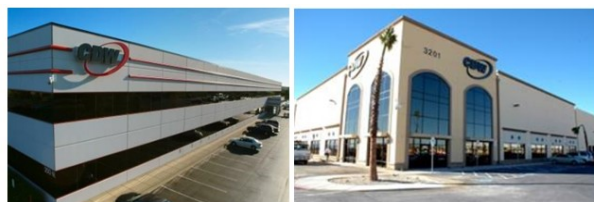
450,000-square-foot distribution center in IL
