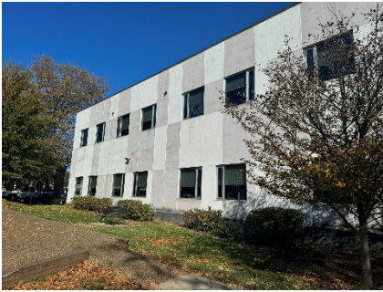
Figure 1: General View of South Elevation towards Student Playground.
