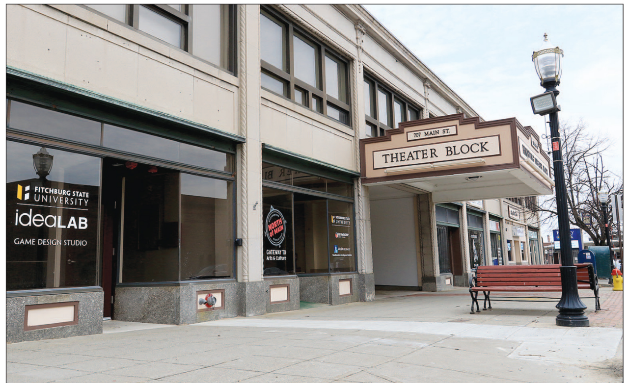
The theater block on Main Street in Fitchburg, where NewVue Communities and Fitchburg State University are working together to help the area's small businesses grow.
