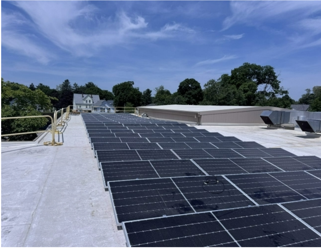
Completed panels on the Middle School roof
