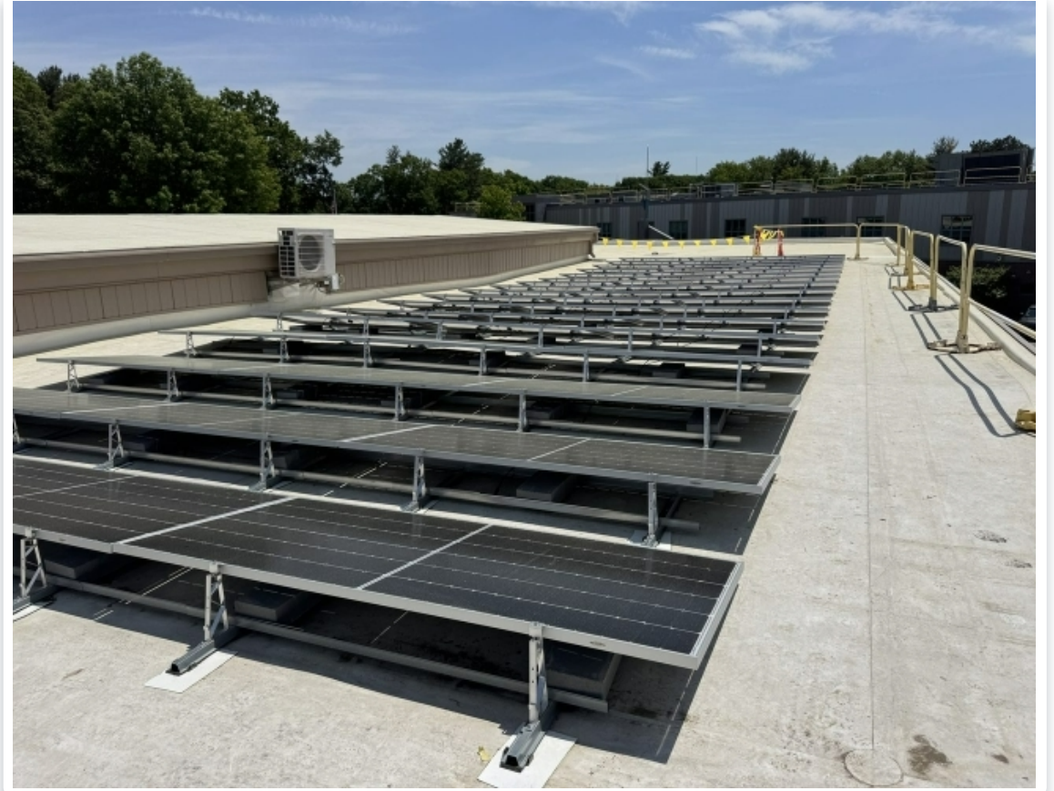
Tilted racking nearing full module layout
