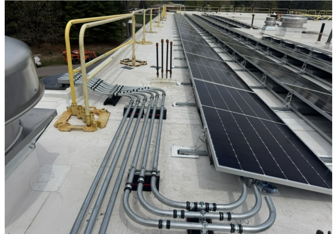
Photos show active equipment and wiring work underway
