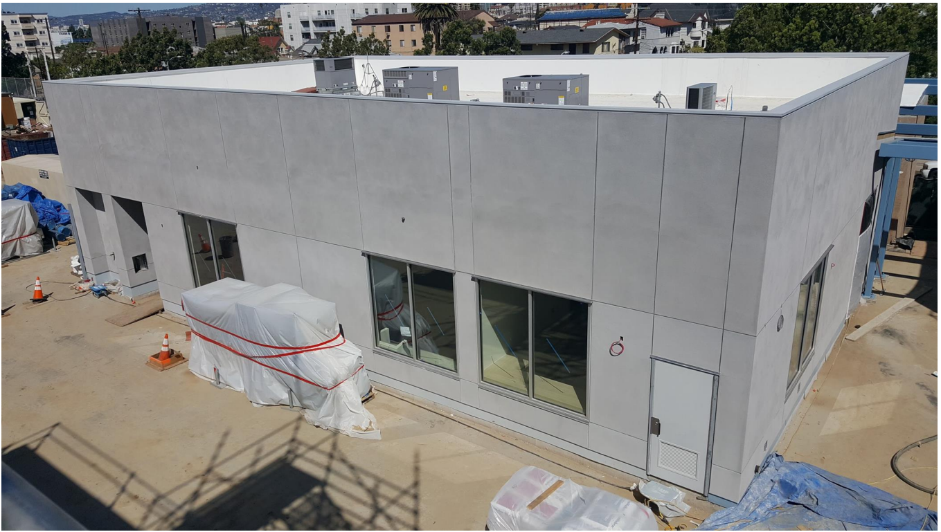
Window glazing installation completed at bldg. A
