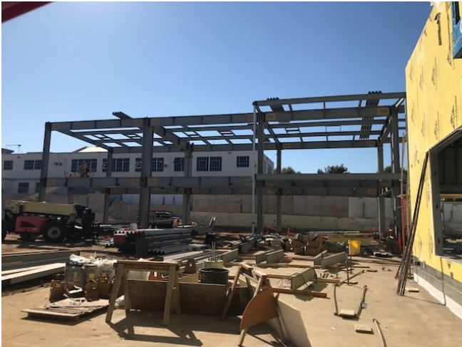
C building Steel (Classroom Building) Administration
