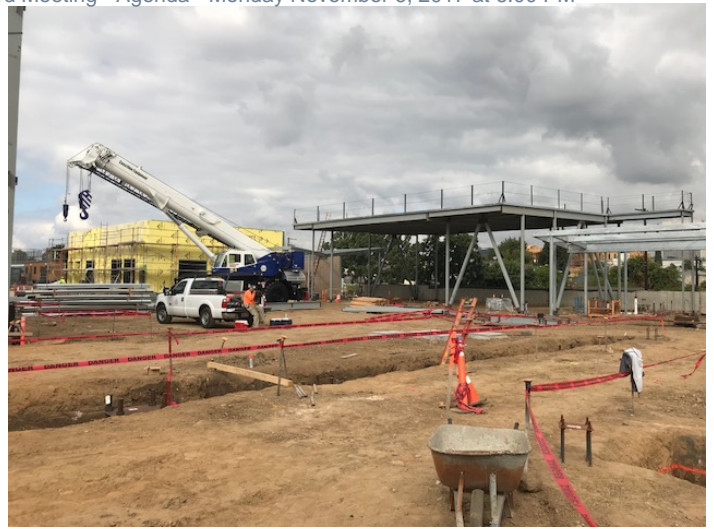
Admin Building, Multi-purpose Room, Lunch Shelter
