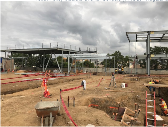
Multi-purpose Room, Lunch Shelter, C building
