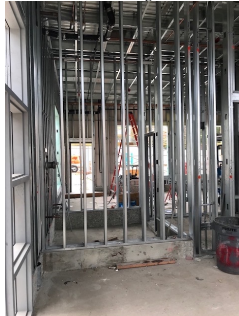
Framing in the Administration Building
