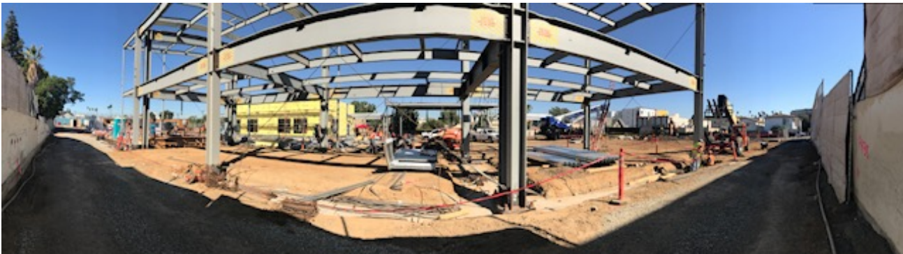
View from the fire lane through the Classroom Building
