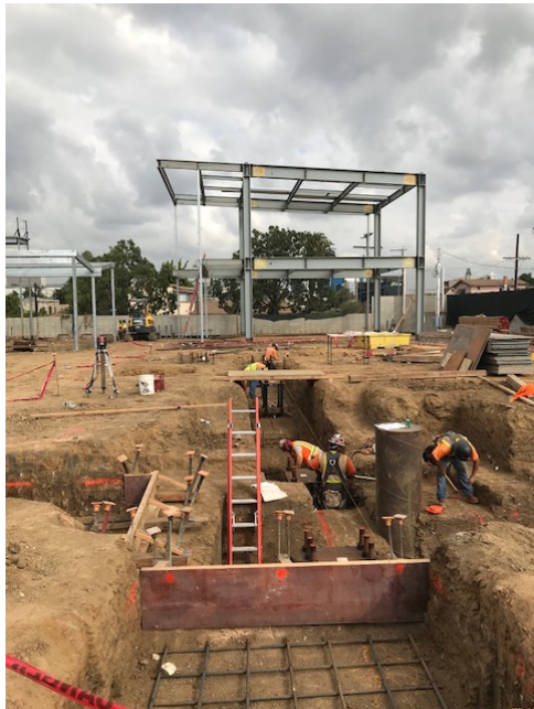
Side of lunch Shelter Elevator Foundation
