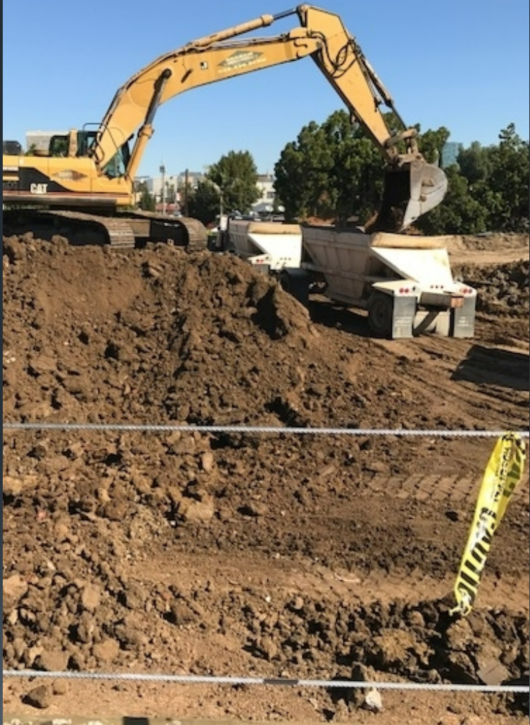
Excavating the underground parking lot
