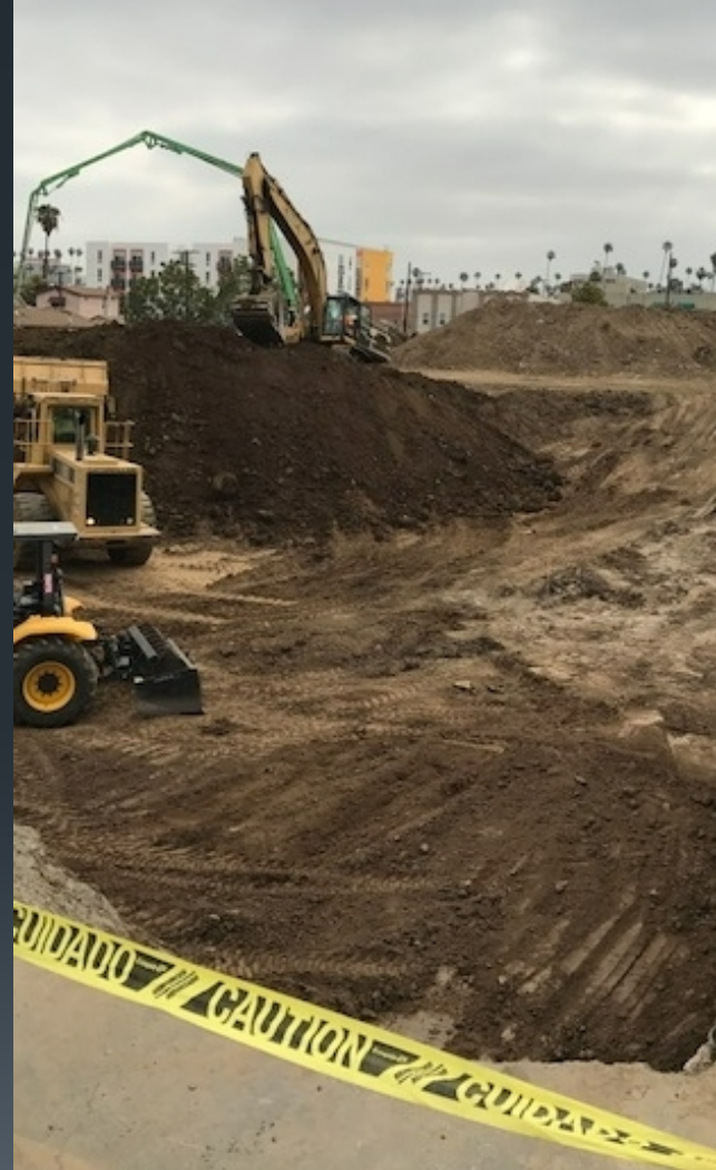
Excavating the underground parking lot
