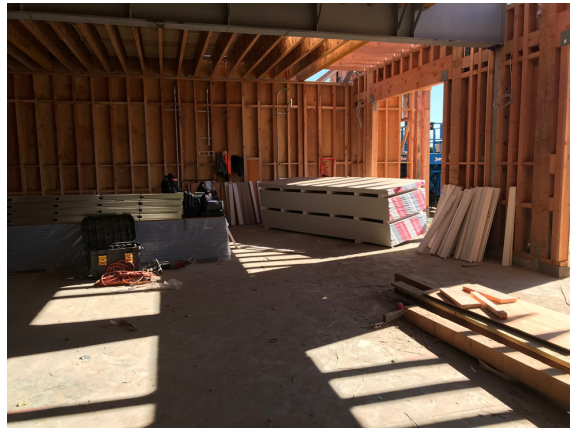
Typical interior construction
