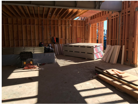
Typical interior construction
