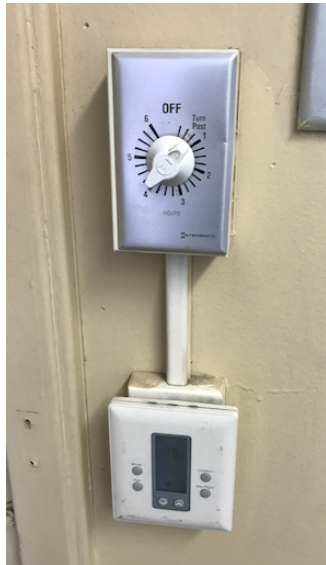
Figure 3: Programmable thermostats w/ 6hr twist timers
