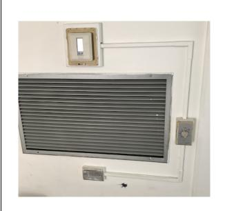
Figure 1: Bard Wall Mounted Heat Pump (4 Ton)
