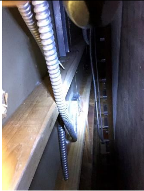
Joists at 2 nd Floor to West Wall
