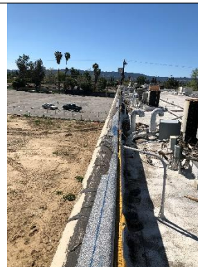
Parapet on East Side After Demo
