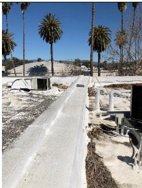
Parapet at West Side Adjacent Building
