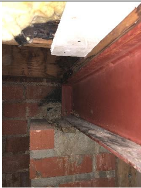
Steel Beam to Pilaster
