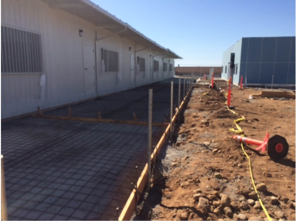
Ready for concrete!
