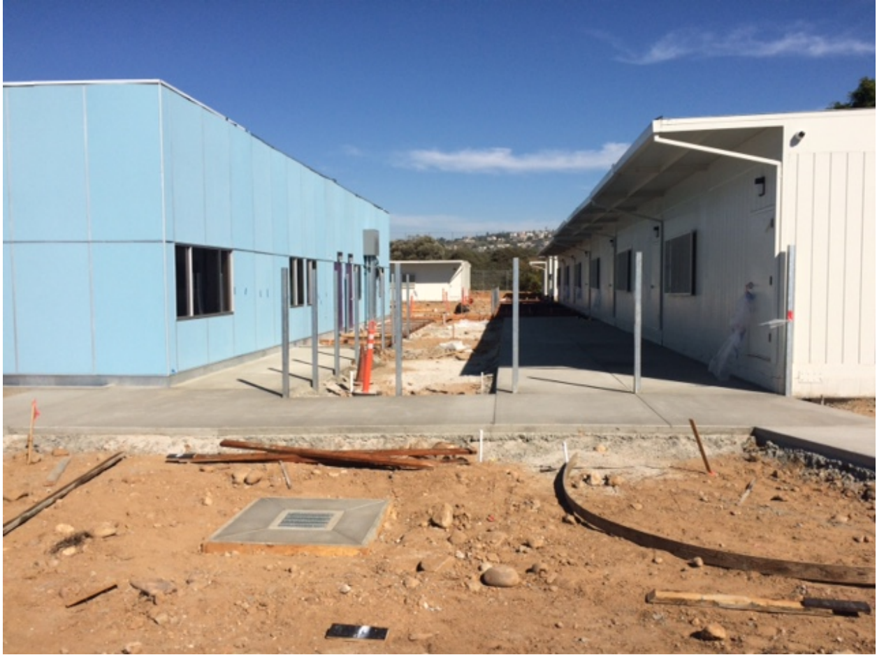
Admin building and classrooms are near ready!
