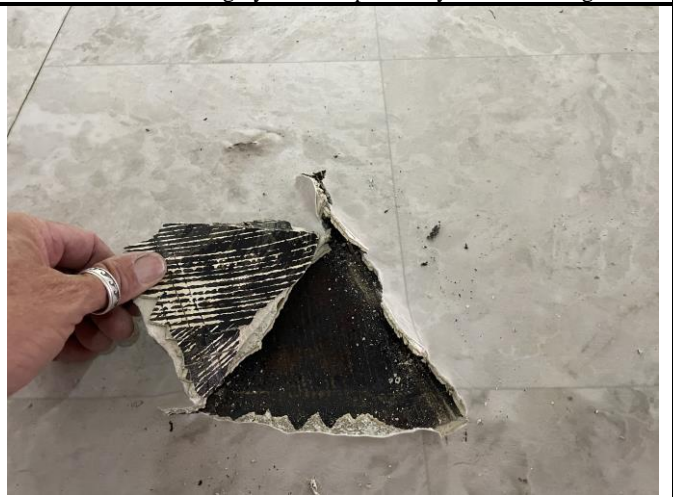
Photo 12: ACM flooring under sheet vinyl
