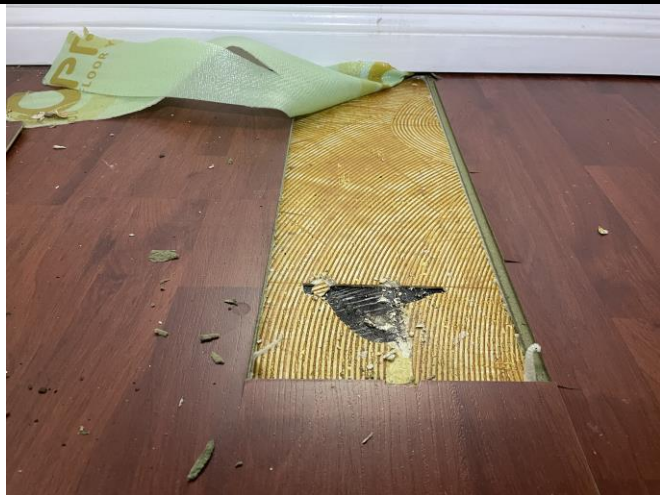
Photo 11: ACM flooring under laminate
