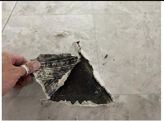
Photo 12: ACM flooring under sheet vinyl
