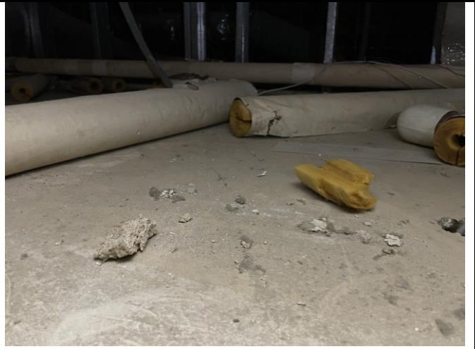
Photo 16: Non-ACM pipe insulation above drop ceiling
