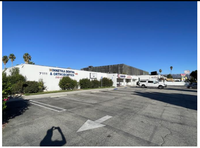
Photo 4: Asphalt paving on the east parking lot
