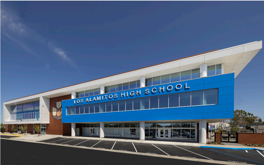
LOS ALAMITOS HIGH SCHOOL STEM BUILDING 3591 Cerritos Ave, Los Alamitos, CA 90720
