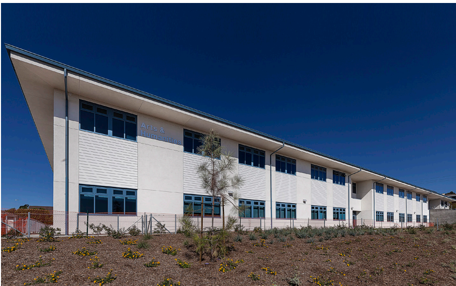
SAN DIEGUITO ACADEMY ARTS & HUMANITIES BUILDING 800 Santa Fe Drive Encinitas CA 92024
