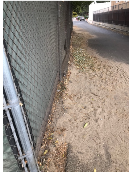
Retaining Wall at Playground
