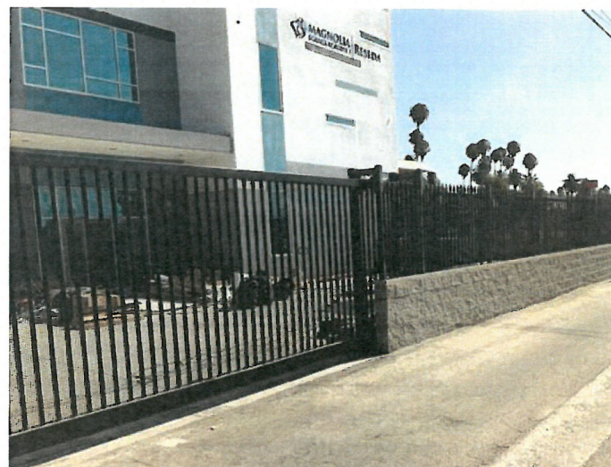
NEW WROUGHT IRON FENCE AT SOUTH PROPERTIES TO MATCH NEW FENCE AT NEW MSA-1 HIGH SCHOOL (PICTURED ABOVE)
