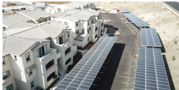
LOCATION Carlsbad, CA STRUCTURE TYPE Semi-Cantilever Structure
