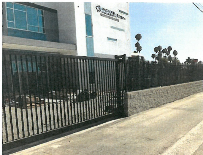
NEW WROUGHT IRON FENCE AT SOUTH PROPERTIES TO MATCH NEW FENCE AT NEW MSA-1 HIGH SCHOOL (PICTURED ABOVE)
