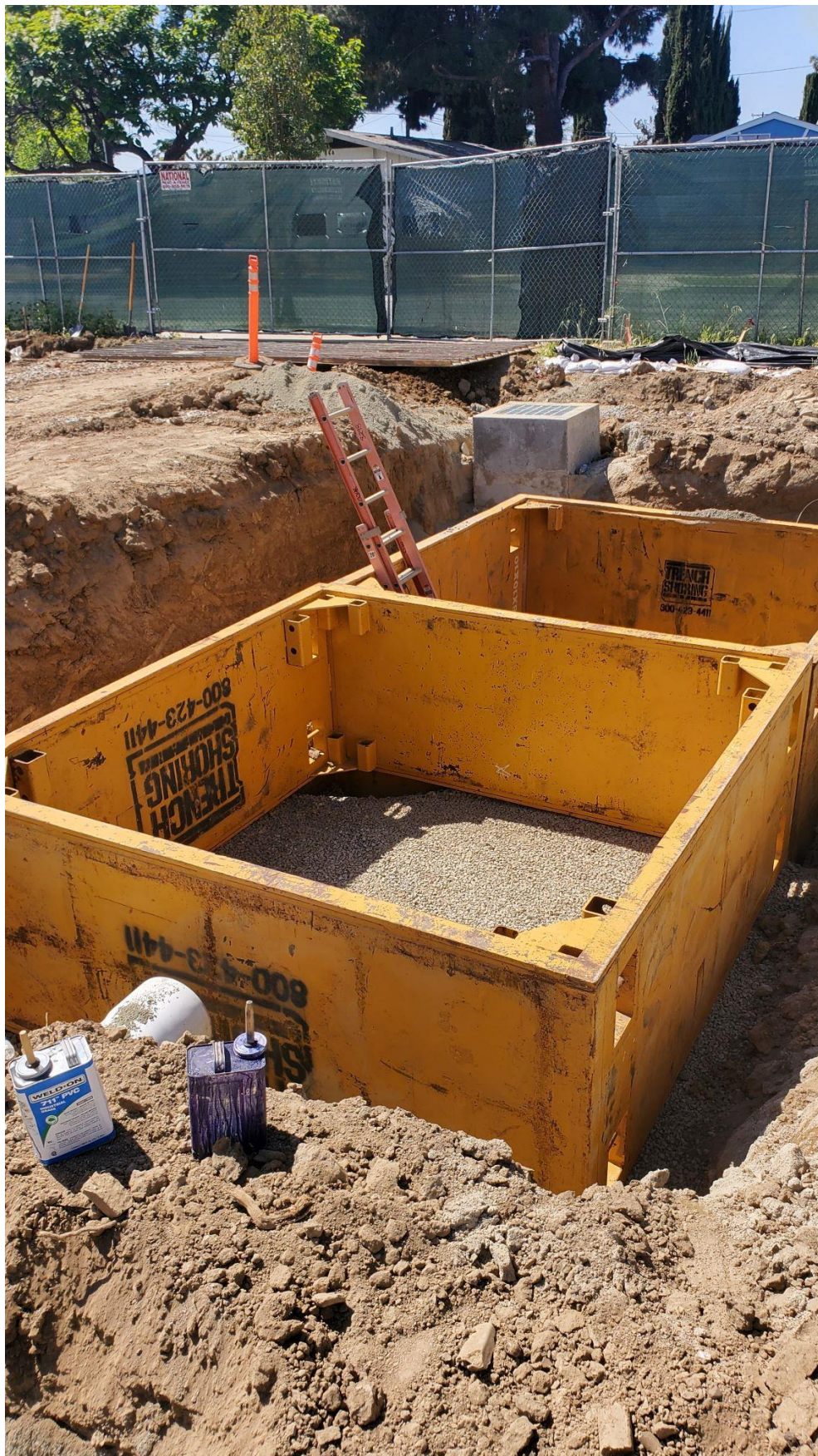
Excavation for Lift Stations w/ Temporary Shoring and Gravel installed
