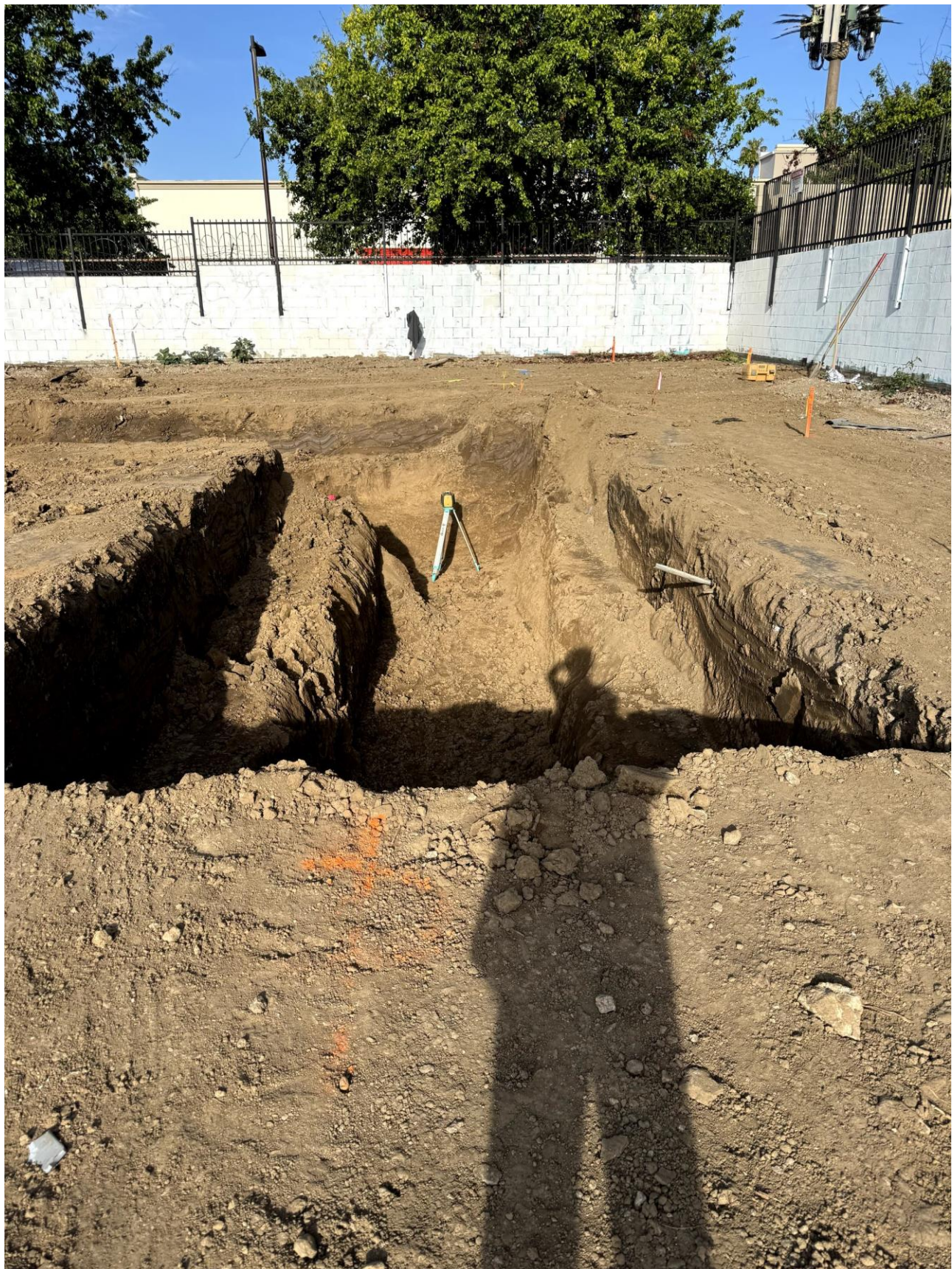
Sewer Line Excavation in Progress
