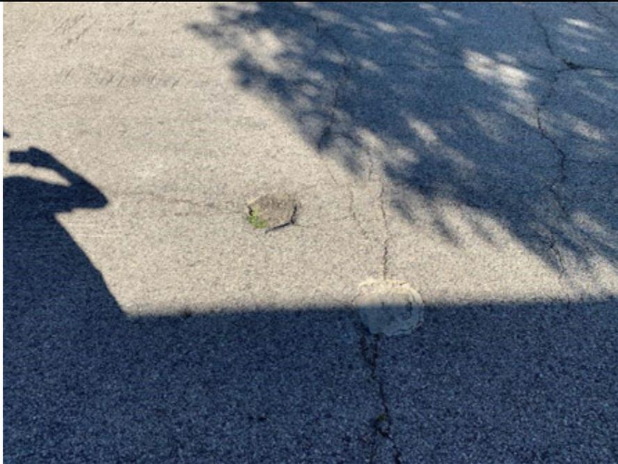
**Photo 9:** View of an 8-inch asphalt patch and a 10-inch concrete patch in the parking lot north of the building on Site.
