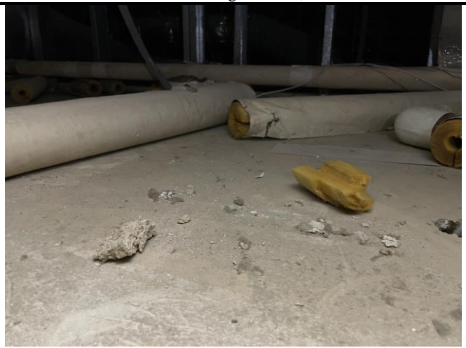
Photo 16: Non-ACM pipe insulation above drop ceiling
