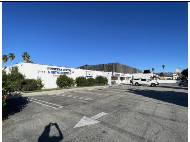
Photo 4: Asphalt paving on the east parking lot
