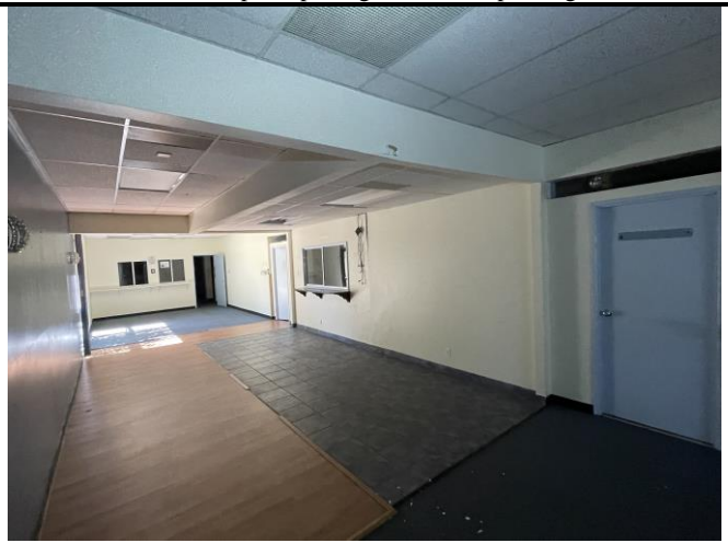
Photo 6: South entrance lobby
