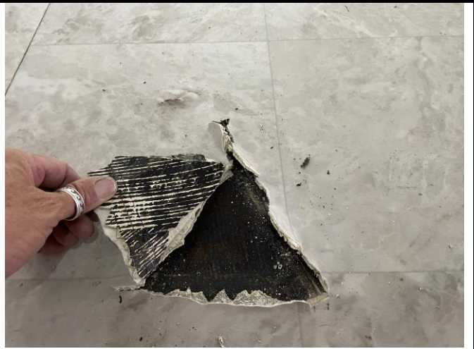
Photo 12: ACM flooring under sheet vinyl
