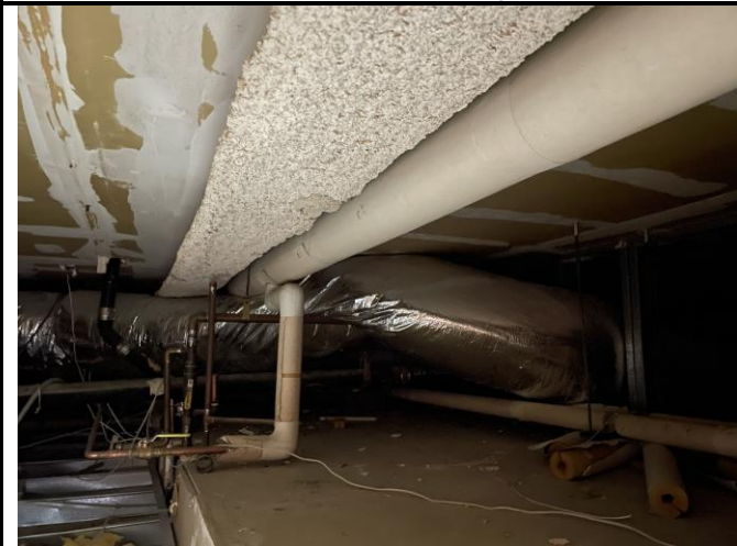
Photo 15: Non-ACM fireproofing on I-Beams above drop ceiling
