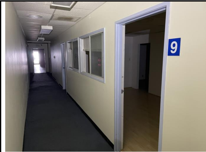
Photo 7: Typical interior corridor
