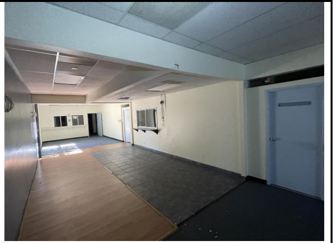
Photo 6: South entrance lobby
