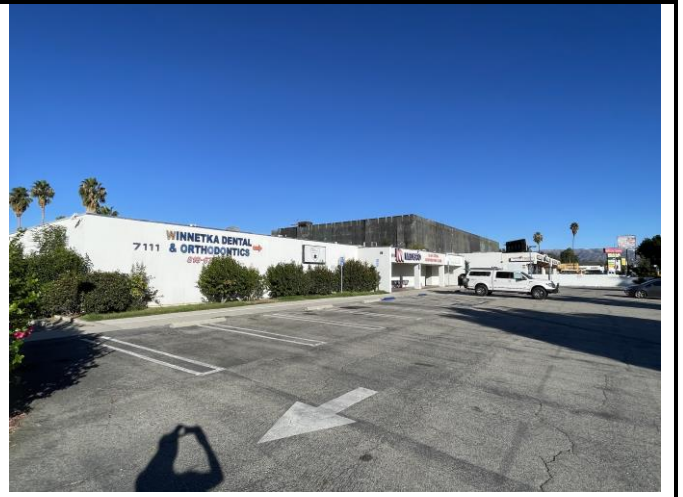
Photo 4: Asphalt paving on the east parking lot
