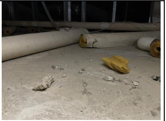
Photo 16: Non-ACM pipe insulation above drop ceiling
