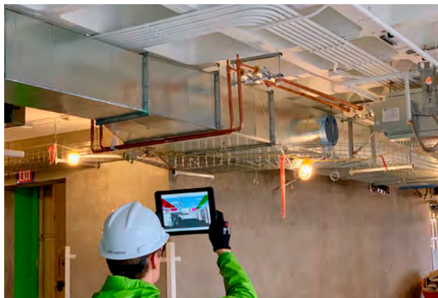
Virtual Reality and other technology can be used to collaborate with the contractor throughout the project, as shown here on a recent project.
