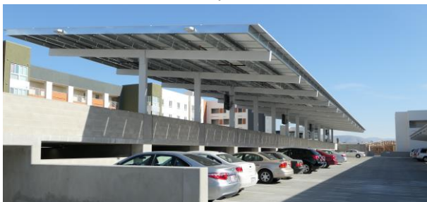
LOCATION Chula Vista, CA STRUCTURE TYPE Parking Garage – “T” Structure
