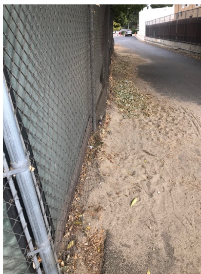
Retaining Wall at Playground
