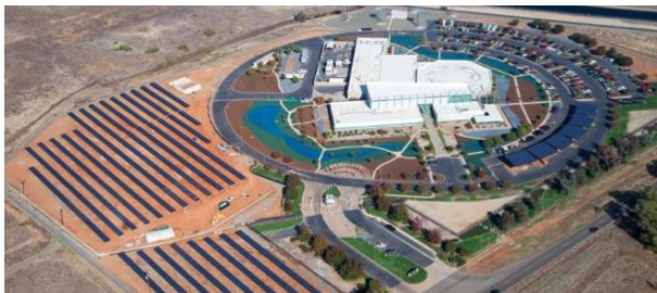
LOCATION Mountain Valley, CA STRUCTURE TYPE Ground Mount & Carports
