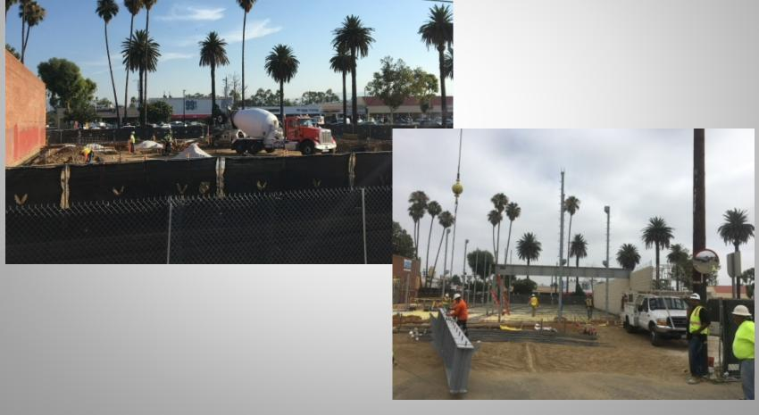
Slab on grade is prepped, placed and done...
