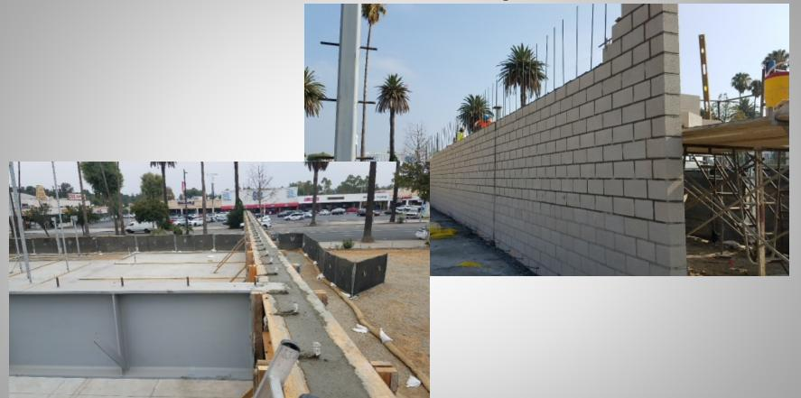
No surprises – completing CMU walls define building exterior on two sides – completing these walls releases the entire building for wood framing
