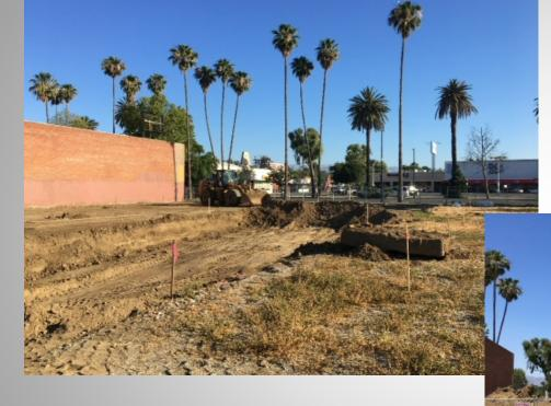
The top 4 feet of soil was removed and re-compacted... work inspected and complete
