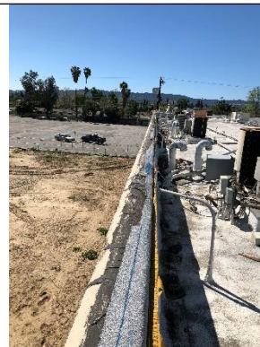
Parapet on East Side After Demo
