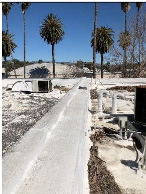
Parapet at West Side Adjacent Building
