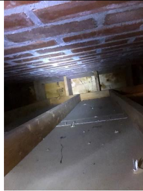
Joists at 2 nd Floor to South Wall
