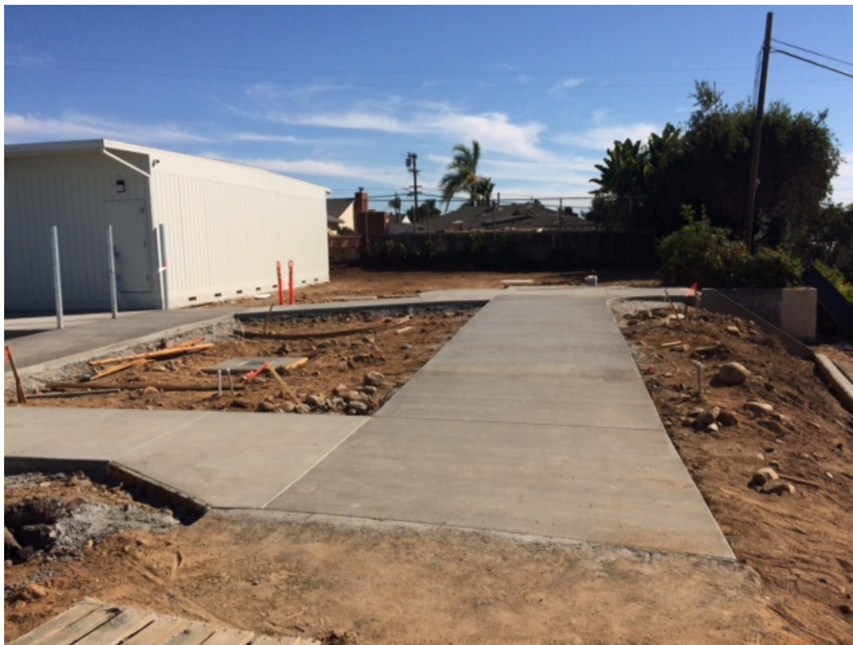
Flatwork and planting beds at front entrance of school. An accessible ramp will be poured in this area.
