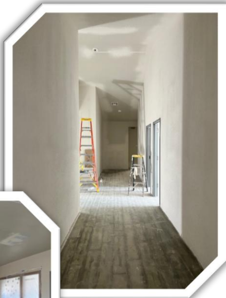
Early Childhood Renovations February
