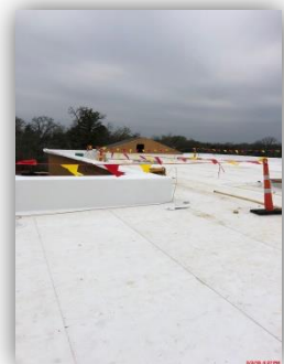
Area A Roof
