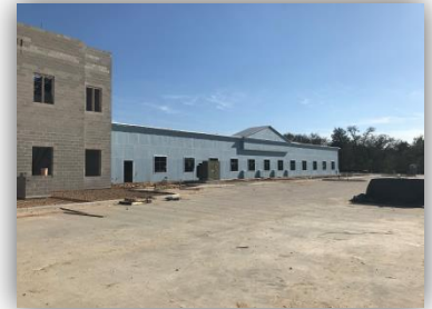
Area A Waterproofing
