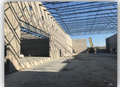
Gym Bar Joists
