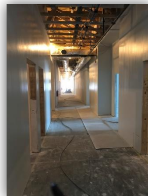
Prime Paint Sheetrock
