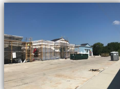
Exterior Progress Area B
