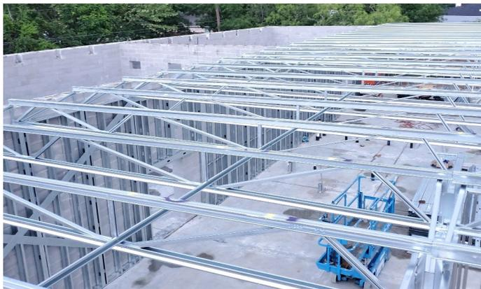
The exterior and structure of the building consists of conventional light gauge metal framing, as well as the truss framing system. This was instigated by Novel and resulted in a significant cost savings.
