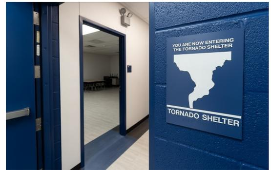
Grand Prairie contains both classrooms and a storm shelter built in full size 12" fully grouted CMU walls. The Storm Shelter is fully self contained with interior water, backup power, and emergency storage.
