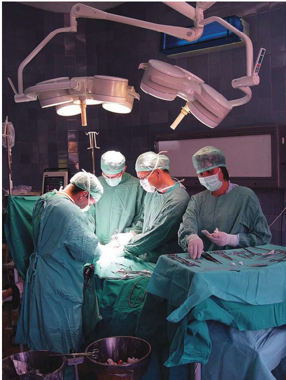
SANITARY SPACE: UV technology, like the glowing blue upper-air fixture on the wall in this surgery room, can reduce the risk of hospital-acquired infections.
